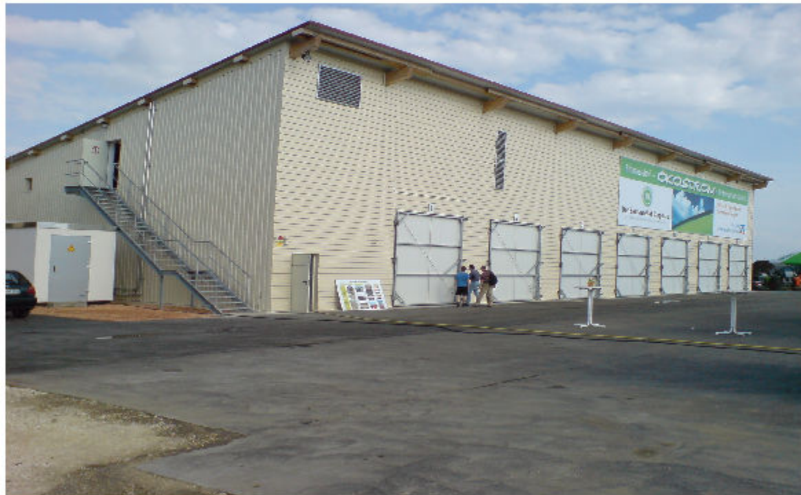
Renergon Dry Fermentation Plant, Langenau, Germany
