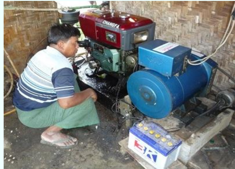
Biogas Engine for electricity production
